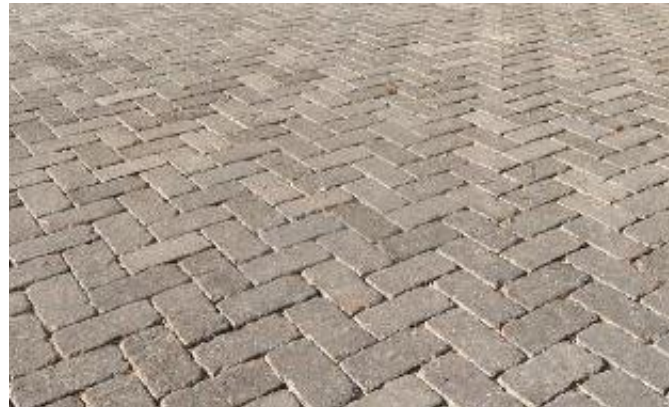
Permeable paving to car park
